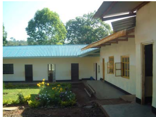
Kilaremo primary school fully renovated
