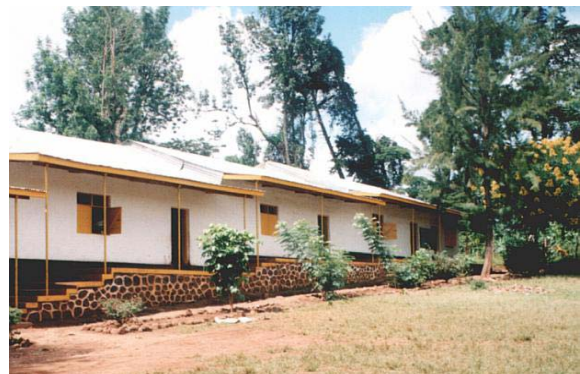
New classrooms at Palangeny
